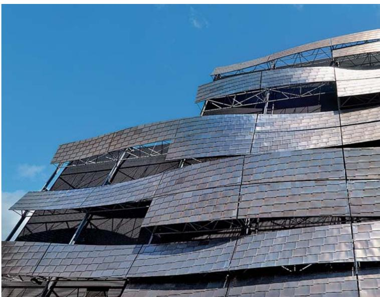
*Each strip of panels is attached to the building structure by a modular set of galvanised-steel frameworks.*
