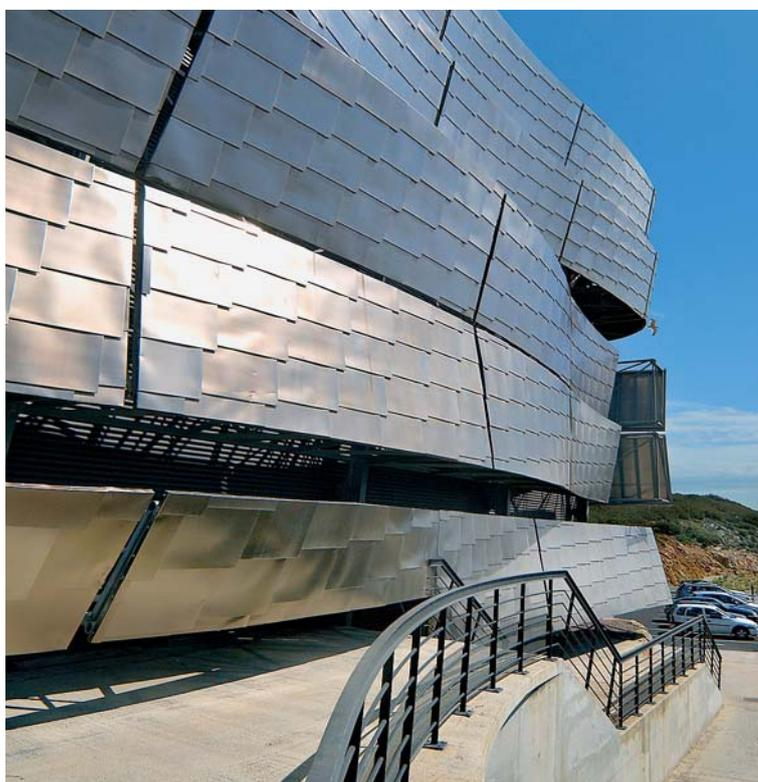
average size of 950 x 600 mm, in collaboration with the architect. These were factory-assembled, to avoid deformation.
